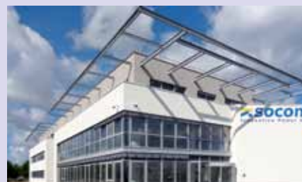
Socomec Green Building.
