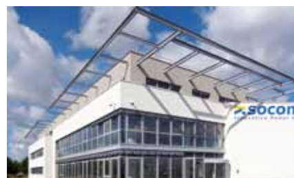
Socomec Green Building.
